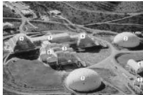
Fig 1.2: [7] Aerial View of Biosphere 2, 1) West Lung, 2) South Lung, 3) Cooling Tower, 4) Energy Center, 5) Intensive Agriculture, 6) Desert, 7) Savannah/marsh, 8) Habitat, and 9) Rainforest
