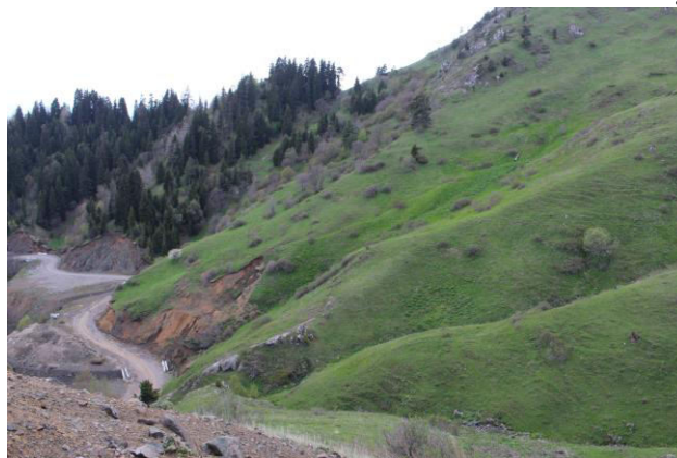
Fig. 7 Avalanche slopes on the Abastumani-Zekari highway, 2023.
