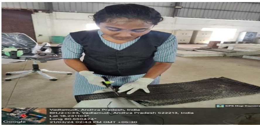
Fig 6Cutting of CFRP sheet
