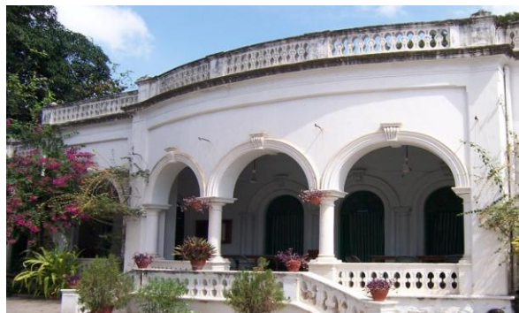
Figure 4 Zenana Mahal, Purani Haveli 1834, notice the semi-circular arches with a prominent key-stone in centre, very European in nature
