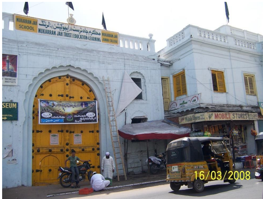
Figure 5 Purani Haveli Palace entrance, notice the Darwaza and Khirki(postern)
