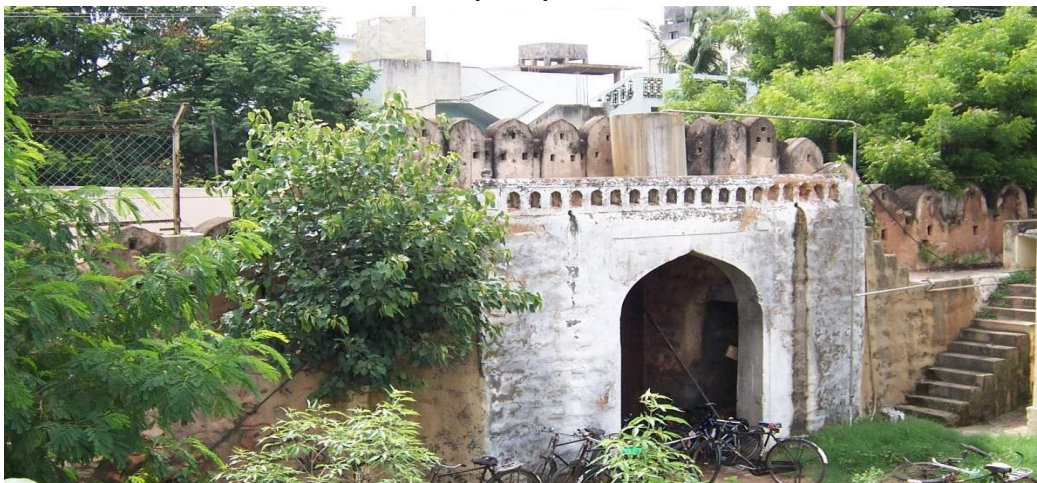
Figure 3 Malkajgiri Baradari, notice the fortified entrance gateway and wall
