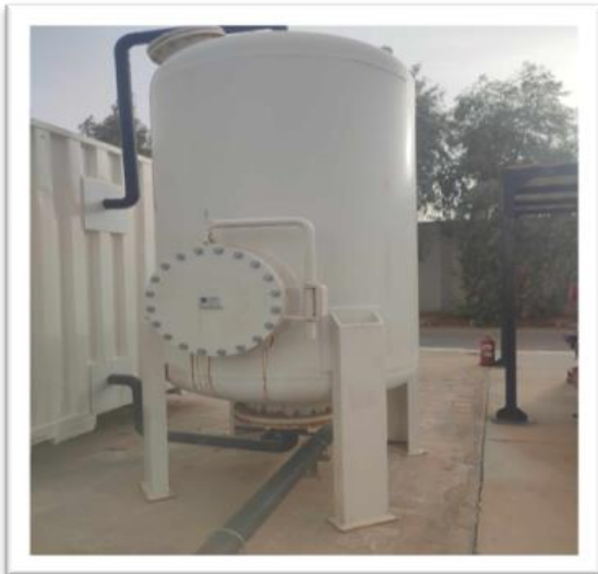
Figure 5: Sand filter
