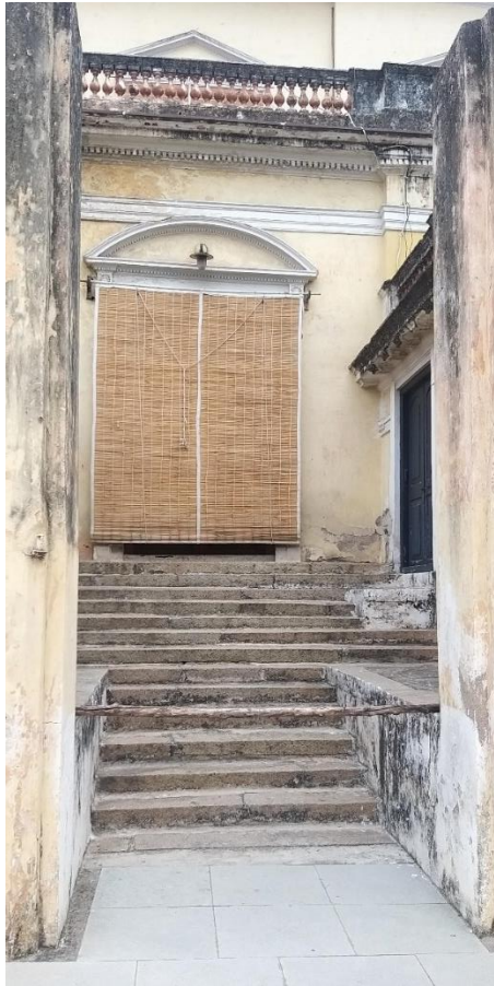
Figure 8 use of natural material to cover the openings is observed in both the palaces also at Domakonda Fort, a very local effort to cool the palace. Picture clicked at Chowmahalla, Afzal Mahal
