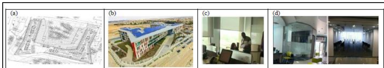
Figure 8:(a,b) Master plan-Perspective shows the building's form based on orientation and the surrounding environment; (c) shading the open office space in the administrative building; (d) Glass walls are used to separate internal spaces.
