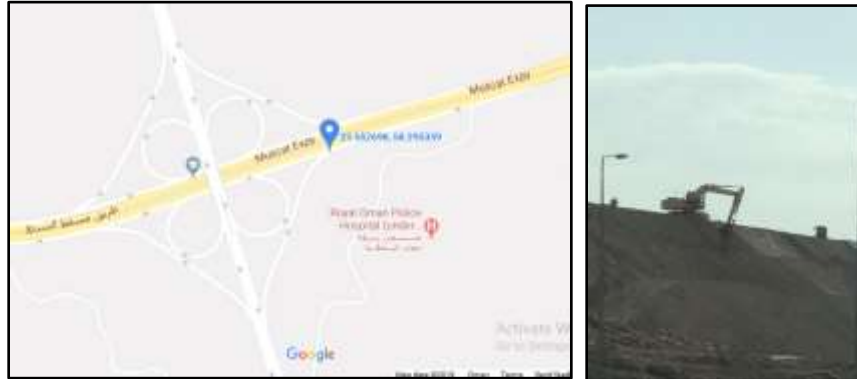
Fig.1 Location of road construction site
